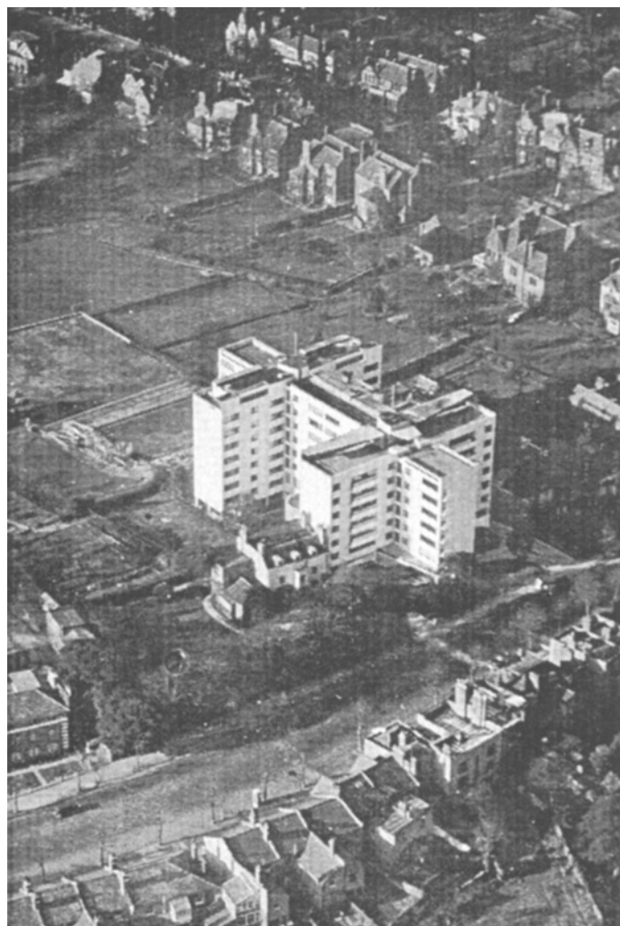
1. Highpoint One, aerial view. (Photo courtesy of John Allan, from Berthold Lubetkin: Architecture and the Tradition of Progress [London: RIBA Publications, 1992].)
